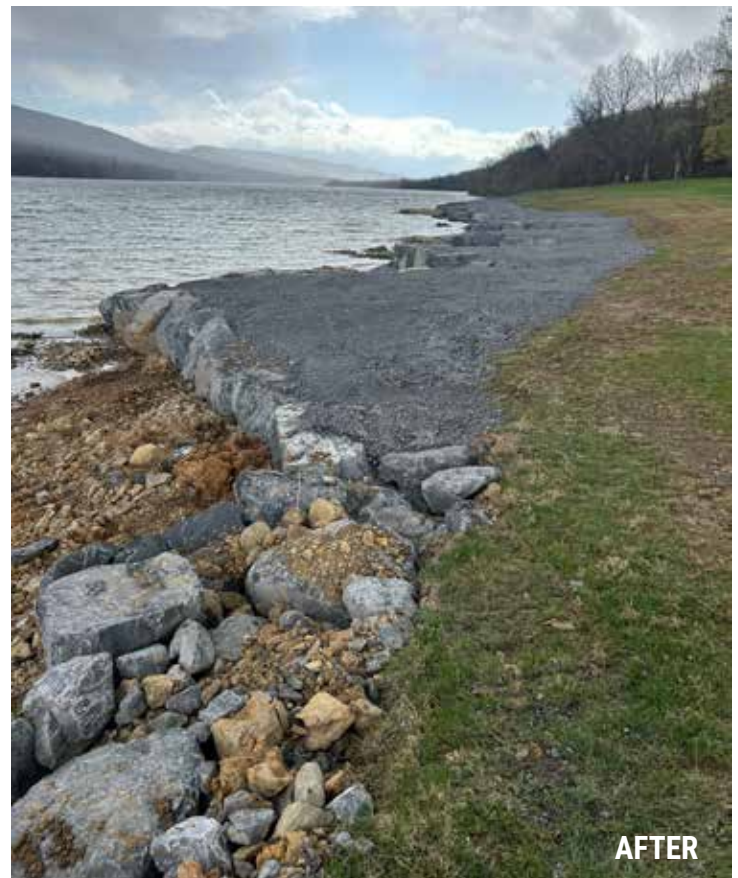
Stone framed deflectors help stabilize the shoreline and prevent further erosion.
