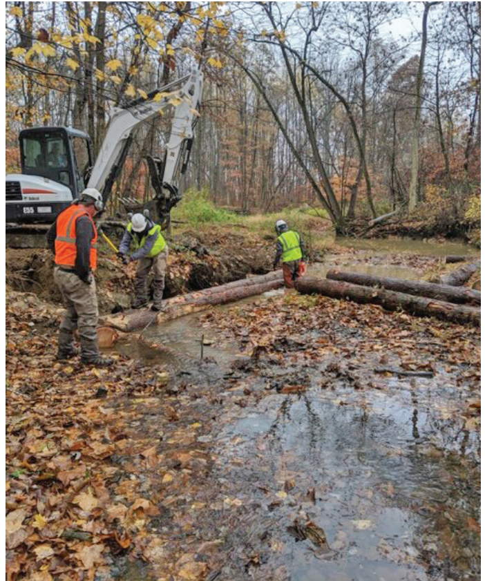
The crew installs mud sills to help stabilize the stream bank at a project site on the West Branch Chillisquaque Creek in Montour County.
