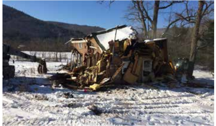
Cavanaugh Access building being demolished.
