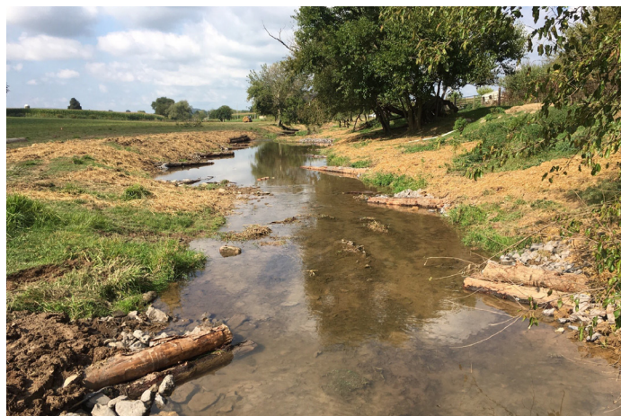
Above: The single log vanes used to stabilize the left stream bank.
