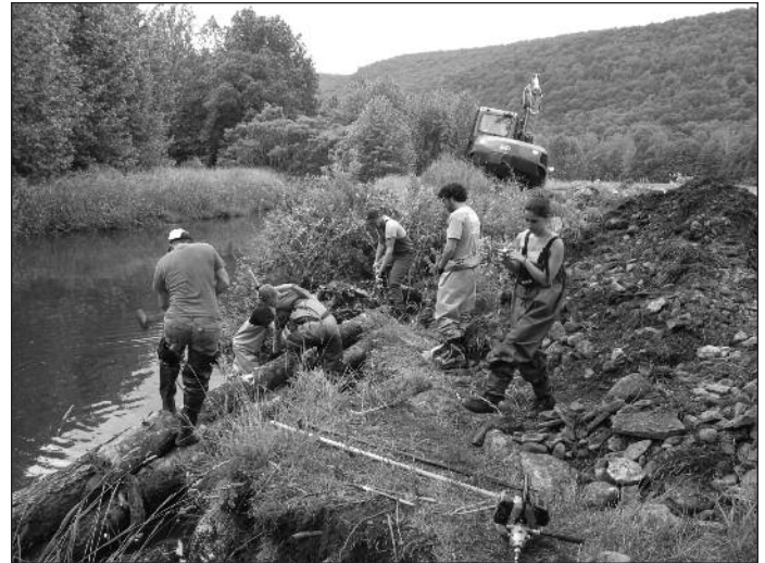
At this project on Wallis Run, interns from Lycoming College worked with PFBC staff to drive rebar. The Loyalsock Creek Watershed Association also had volunteers on hand during this project.
