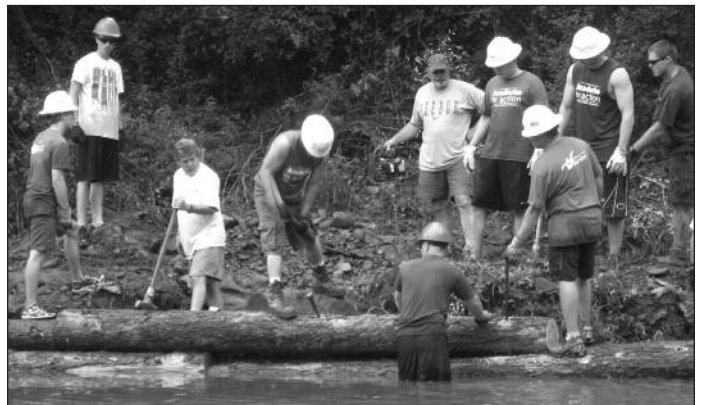
Installing in-stream habitat structures
